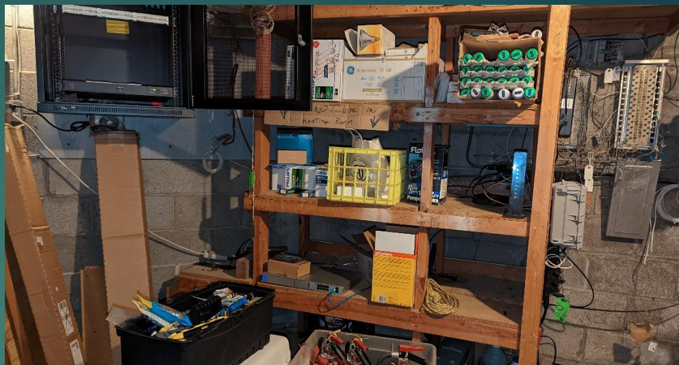
Above: Rack with networking equipment being installed
